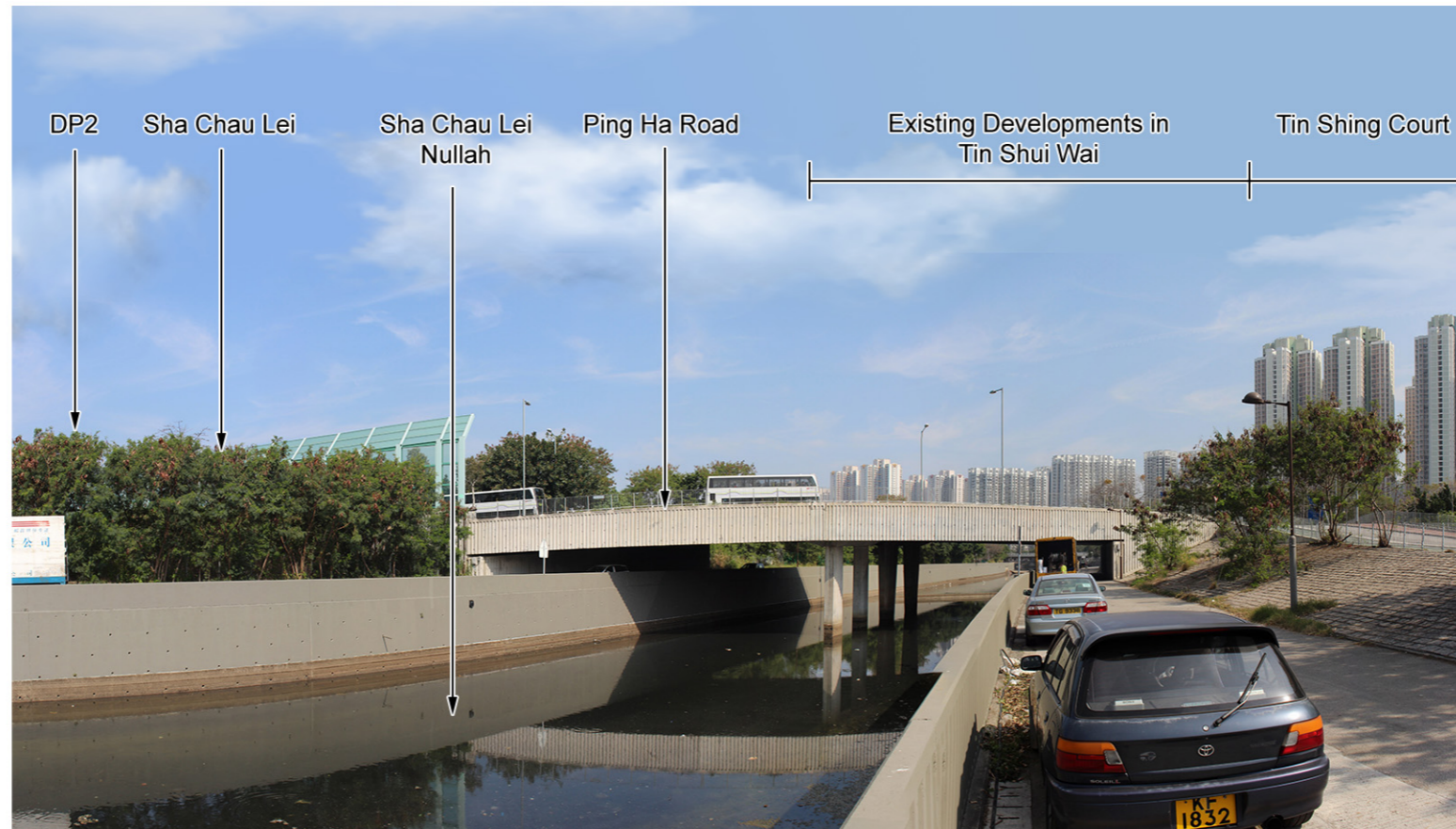
Existing Baseline Conditions
