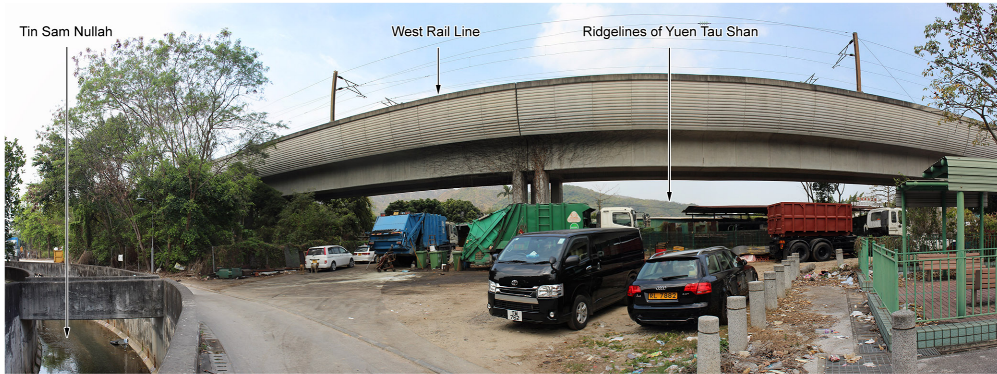
Existing Baseline Conditions
