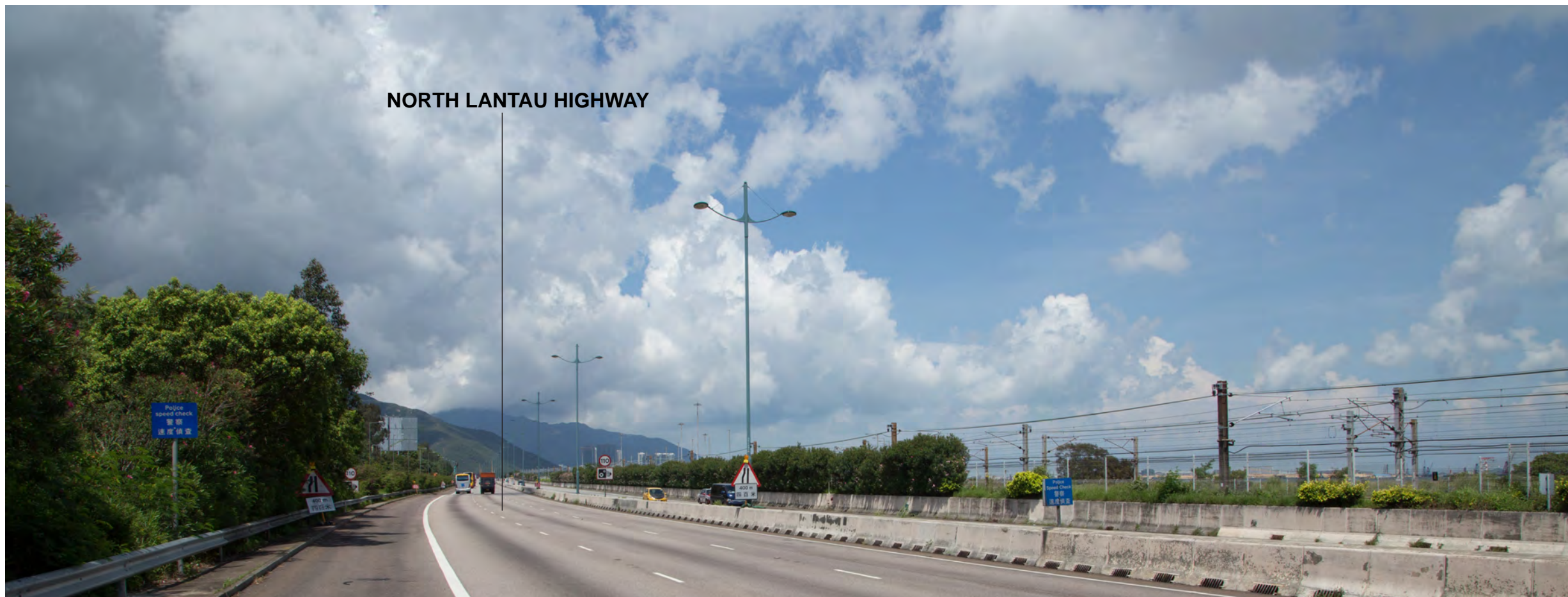
VSR8 North Lantau Highway - Existing View (Approx. 275m)
