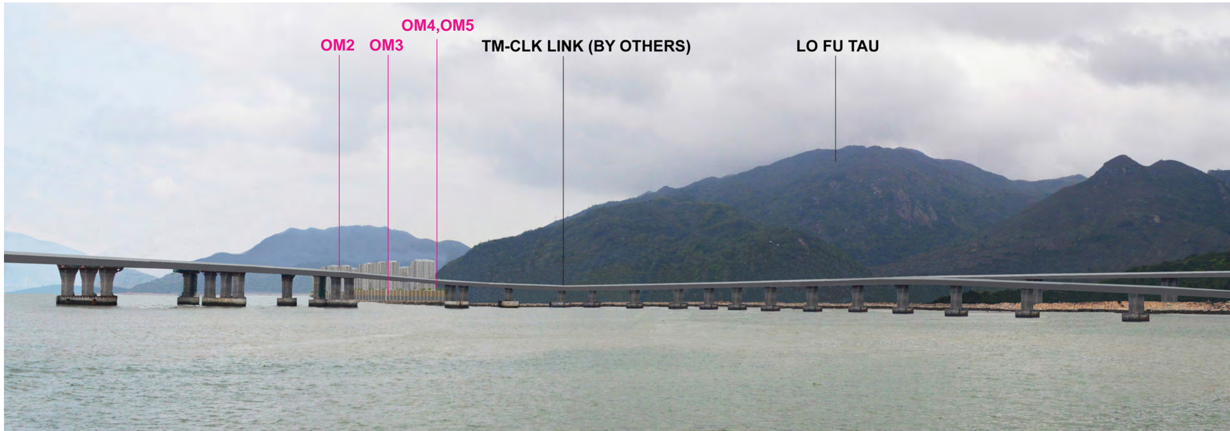
VSR1 Tung Chung New Town Extension Tung Chung East Development (TCNTE TCE Development) - Photomontage (With mitigation at Day 1)
