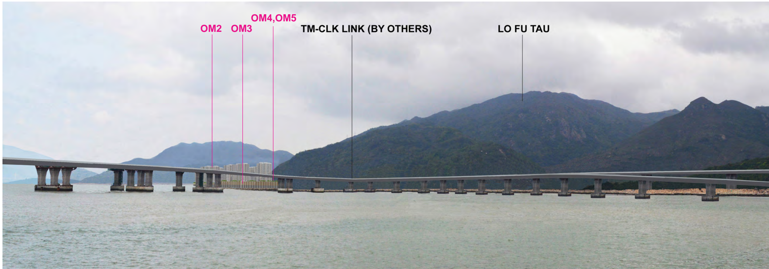
VSR1 Tung Chung New Town Extension Tung Chung East Development (TCNTE TCE Development) - Photomontage (With mitigation at Year 10)
