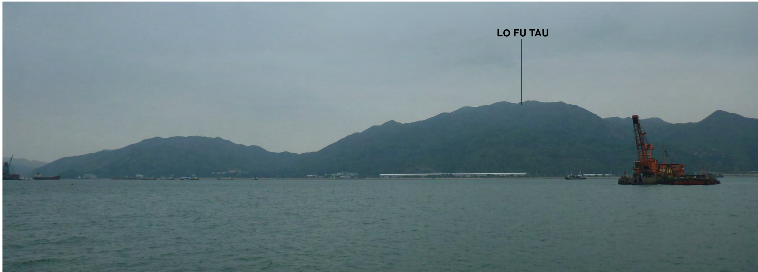
VSR6 Hong Kong Boundary Crossing Facilities - Existing View (Approx. 2390m)
