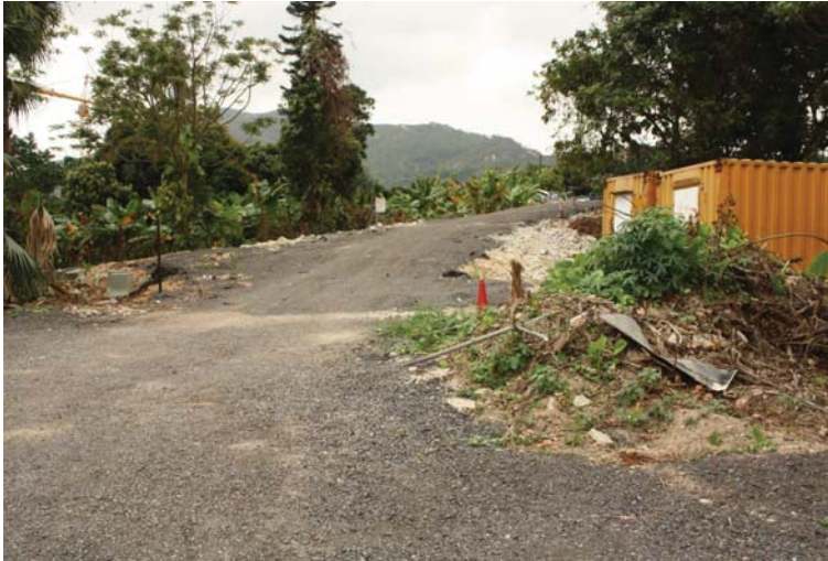
Plate B.1 A new road being constructed.
