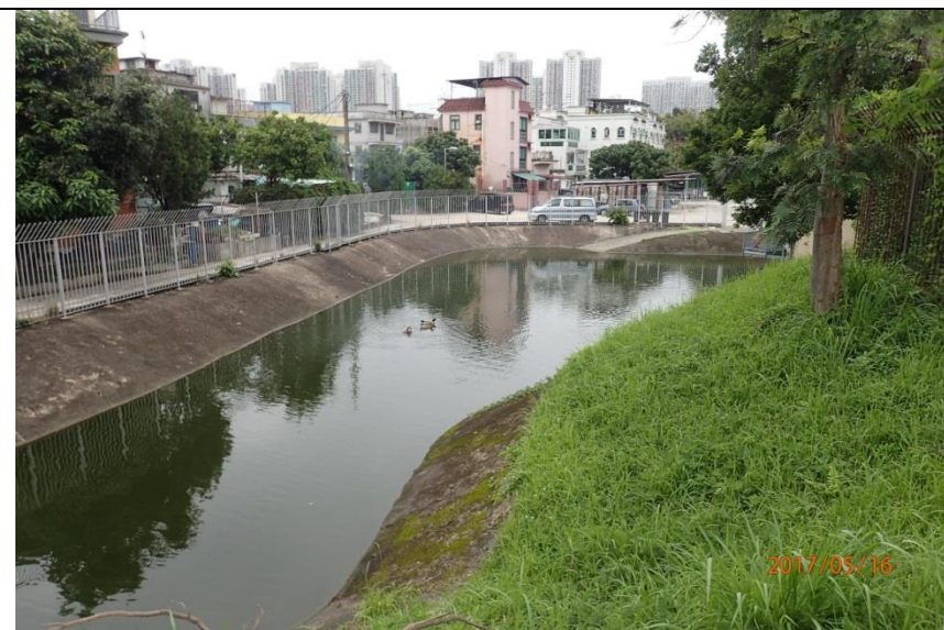
Sik Kong Tsuen Stormwater Pumping Station (Pond #50)
