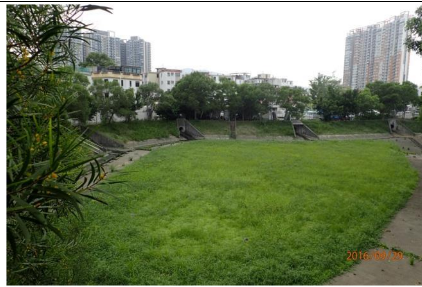
Ma Tin Tsuen Stormwater Pumping Station (Pond #39)
