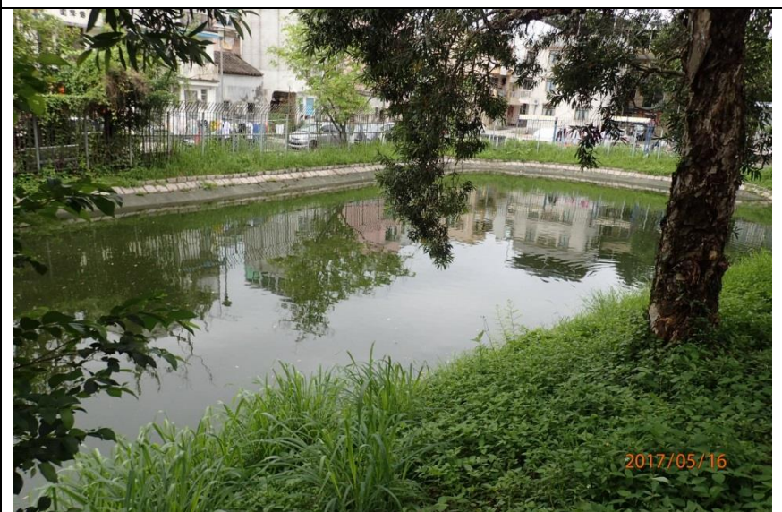
Sik Kong Wai Stormwater Pumping Station (Pond #49)
