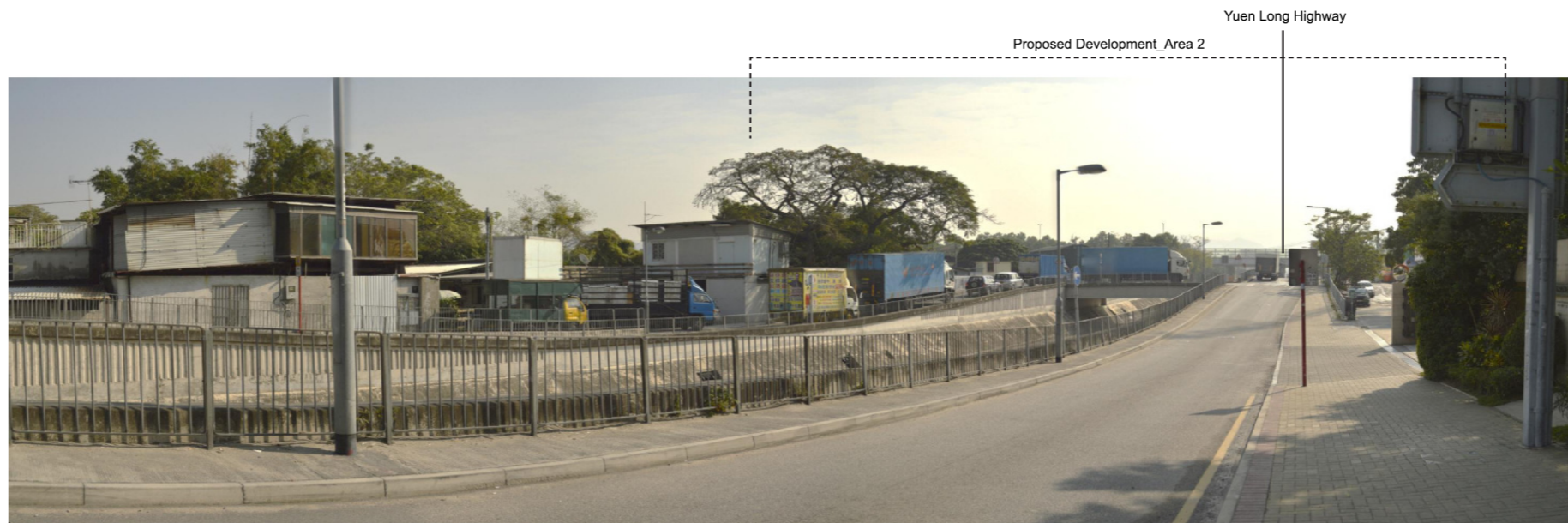
VSR9 Intersection of Kung Um Road and Shap Pat Heung Road
