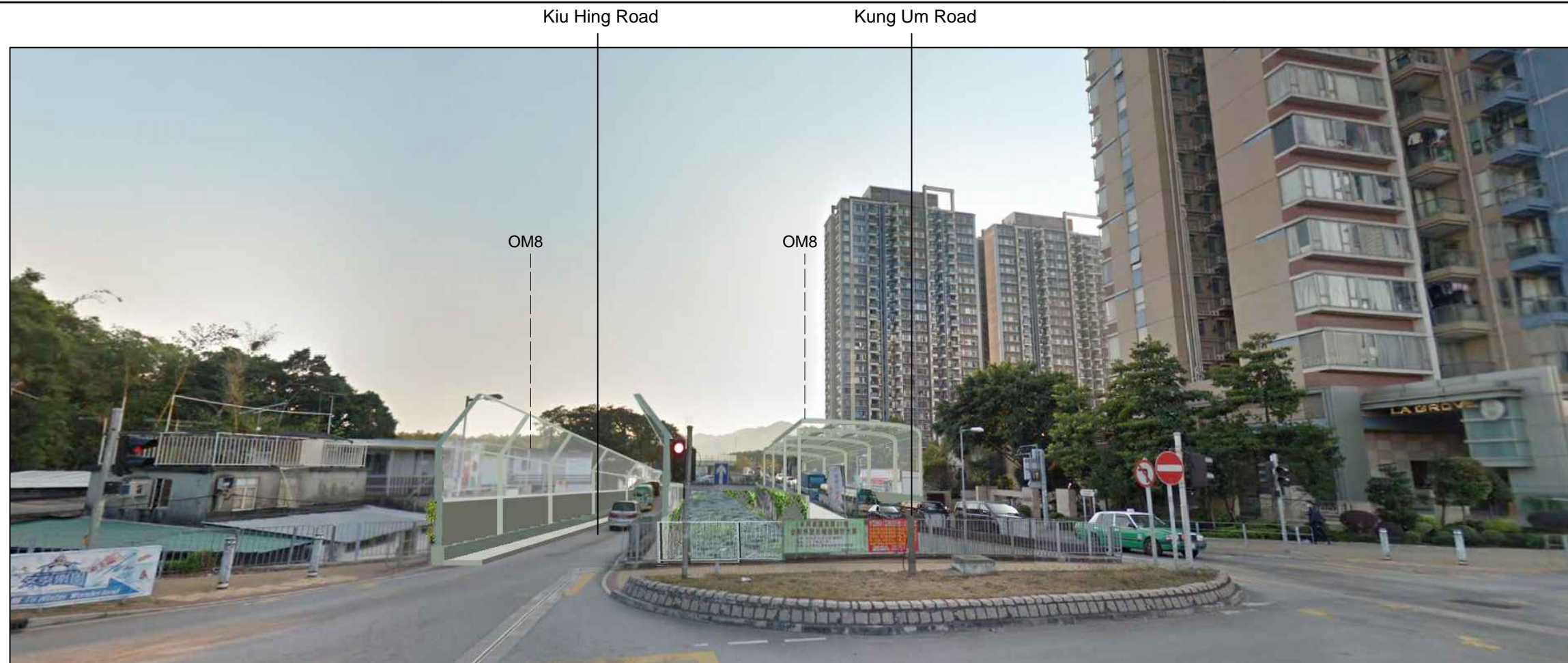
VSR44 Shap Pat Heung Road near La Grove - Photomontage (With mitigation at Day 1)
