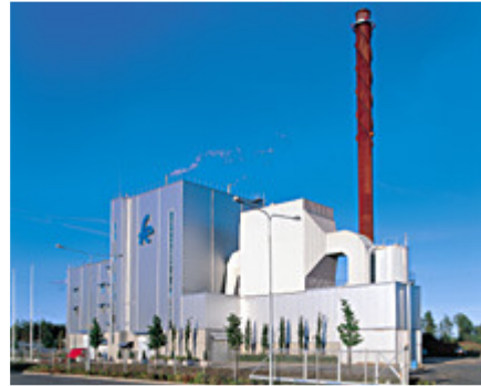
Biofuels station in Finland 261
