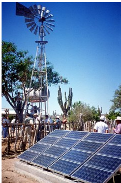
Application of photovoltaic 431
