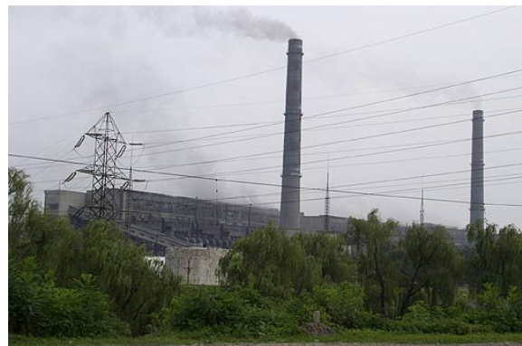
Power plant in Korea 65
