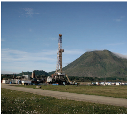
Kawerau Geothermal power station 139
