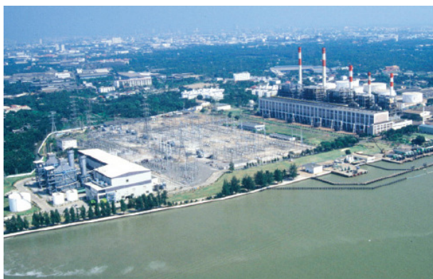
Power Plant in Thailand 75
