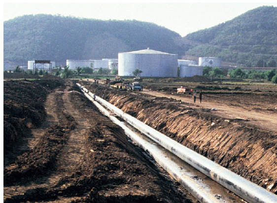
Laying of Natural Gas Pipelines 76
