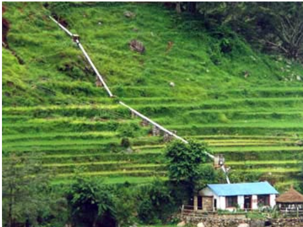
Power house in rural area 448
