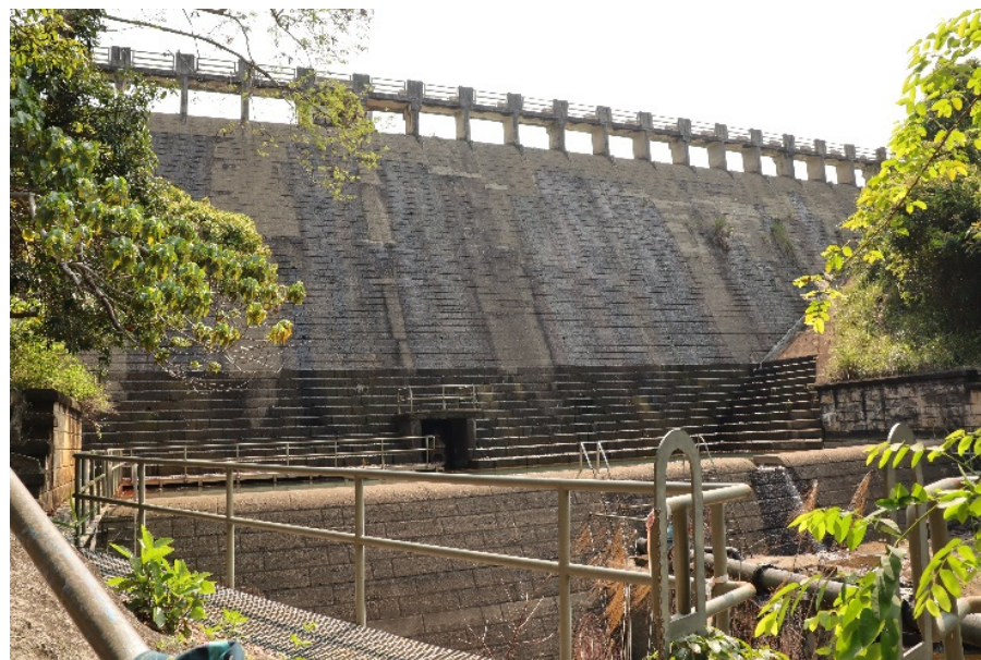
DM-01 - Aberdeen Lower Reservoir, Dam DM-01 - 香港仔下水塘水壩
