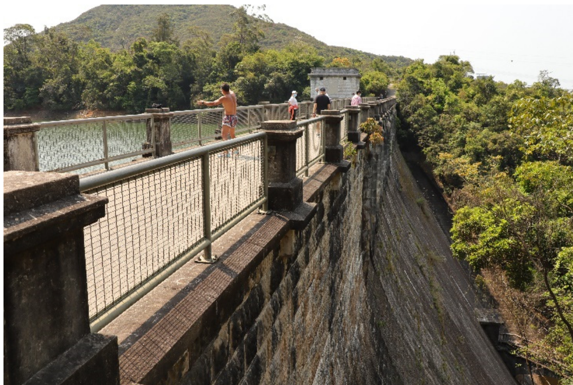
DM-02 - Aberdeen Upper Reservoir, Dam DM-02 - 香港仔上水塘水壩
