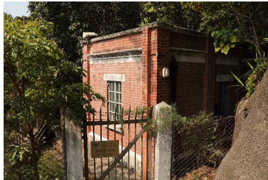
GB-01 - Aberdeen Reservoir, Lower Reservoir, Pump House GB-01 - 香港仔水塘下水塘泵房
