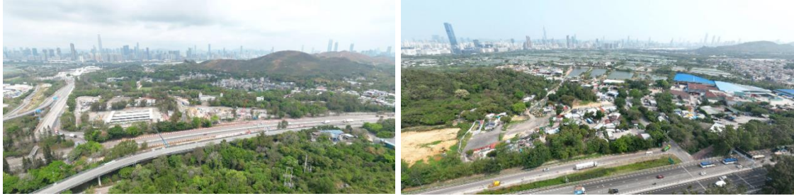
Northern Project Area at the north of San Tin Highway and Fanling Highway
