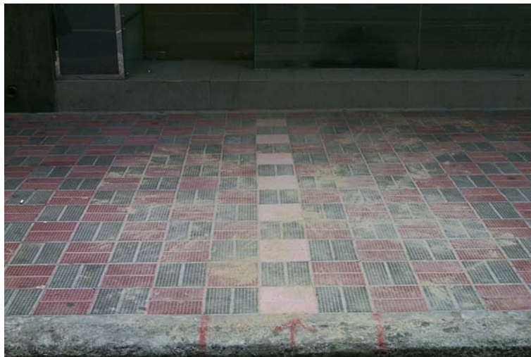
[Picture 2] Blocks were paved across a pedestrian walkway.
