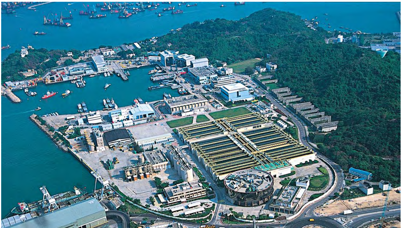
Stonecutters Island Sewage Treatment Works is the largest of its kind in the world
