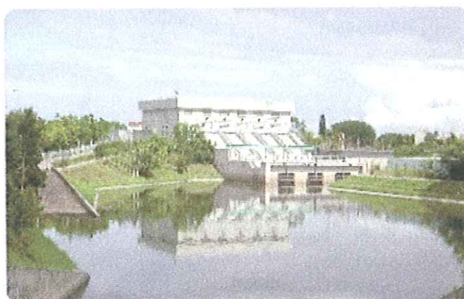
Chuk Yuen Floodwater Pumping Station
