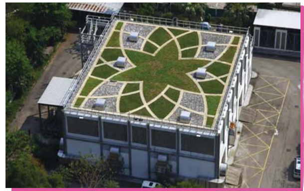
Green roof at Ma On Shan Sewage Pumping Station
