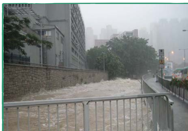
Flooding at Kai Tak Nullah
