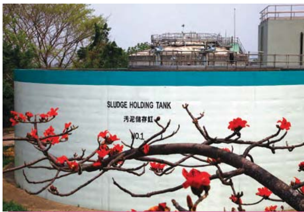
Sludge holding tank at Yuen Long Sewage Treatment Works
