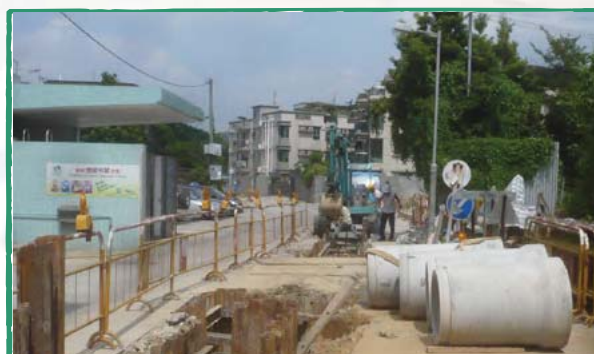
Sewerage under construction at Wing Ning Tsuen, Fanling
