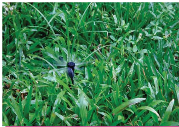
Reclaimed water for irrigation at Shatin STW
