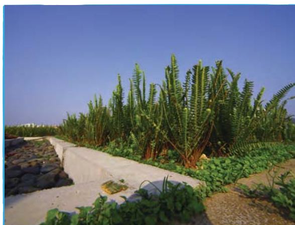
Plants on green roof at Shatin Sewage Treatment Works
