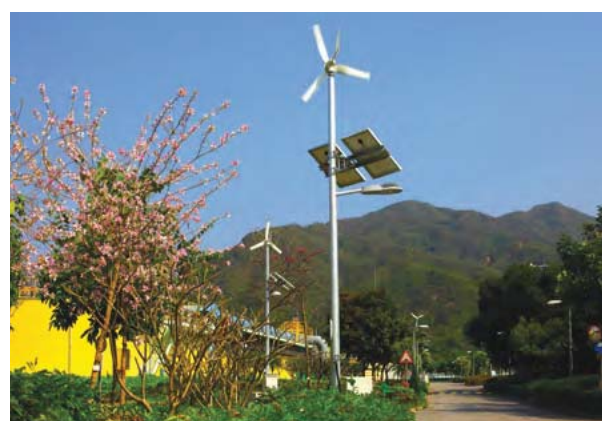
Solar-wind power lamp poles at Shatin STW
