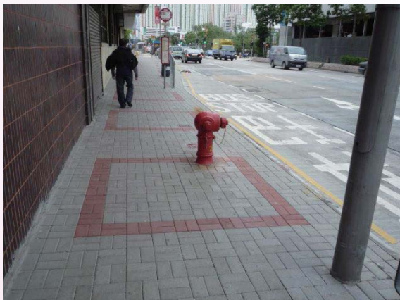
Paving blocks with recycled glass at Wang Kwong Road
