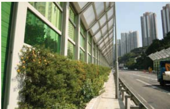
Green walls/noise barriers along Tseung Kwan O Road
