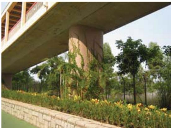
Footbridge across Wetland Park Road, Tin Shui Wai (NF 383)
