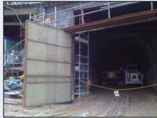
Acoustic Enclosure is under preparation for tunnel works at the magazine site
