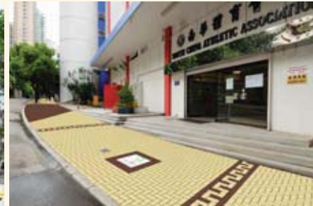
Footway at Caroline Hill Road
