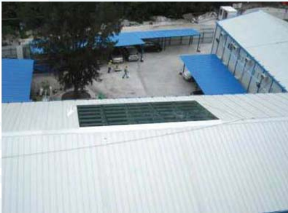
Skylight system at CRE's office
