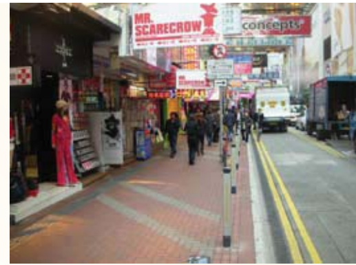
Footpath reconstruction works at Lockhart Road
