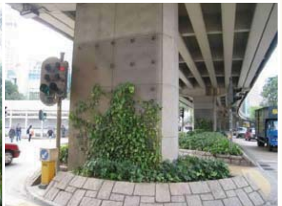
Gascoigne Road Flyover at Gascoigne Road near Wylie Road (K37)
