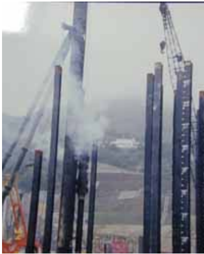
Phasing out of diesel hammer percussive piling with more environmentally friendly mini-piles to reduce air and noise pollution
