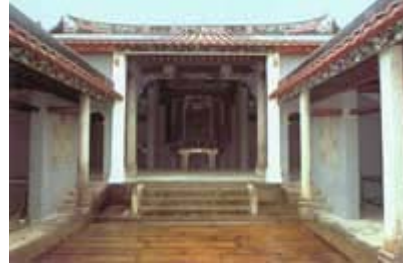
Cheung's Ancestral Hall (after restoration) in Shan Ha Tsuen, Yuen Long
