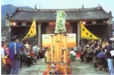
Restoration work for Tang's Chung Ling Ancestral Hall - Lung Yeuk Tau Heritage Trail in Fanling
