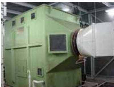
Water scrubber system to reduce odour nuisance
