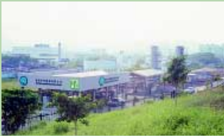
Landfill gas recovered from an old landfill is utilised in the nearby town gas plant
