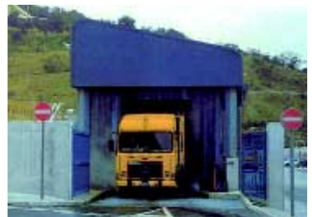
Waste vehicles are thoroughly washed before leaving the refuse transfer station
