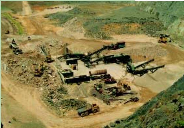
Construction and demolition materials from the waste delivered to the SENT landfill are sorted out for beneficial use
