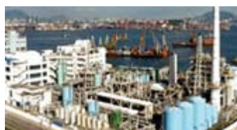
Tsing Yi Chemical Waste Treatment Centre
