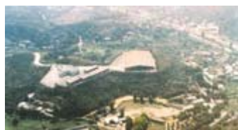
Sha Ling Livestock Waste Composting Plant
