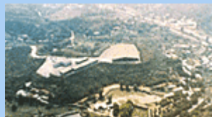
Sha Ling Livestock Waste Composting Plant
