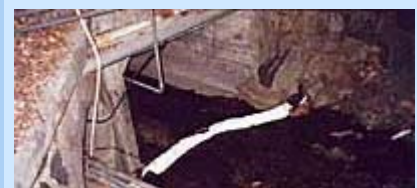
Oil boom used to prevent oil slick from spreading
