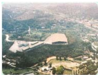
Sha Ling Livestock Waste Composting Plant
