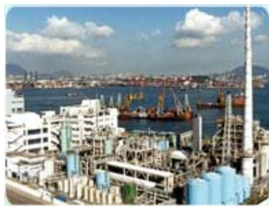
Tsing Yi Chemical Treatment Centre
