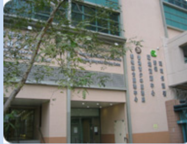
Fanling Environmental Resource Centre.
