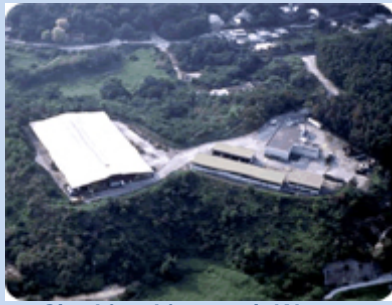
Sha Ling Livestock Waste Composting Plant.
