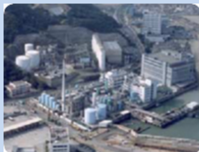
Chemical Waste Treatment Centre, Tsing Yi.
