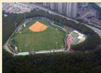
Sai Tso Wan Recreation Ground. (Restored Sai Tso Wan Landfill)
