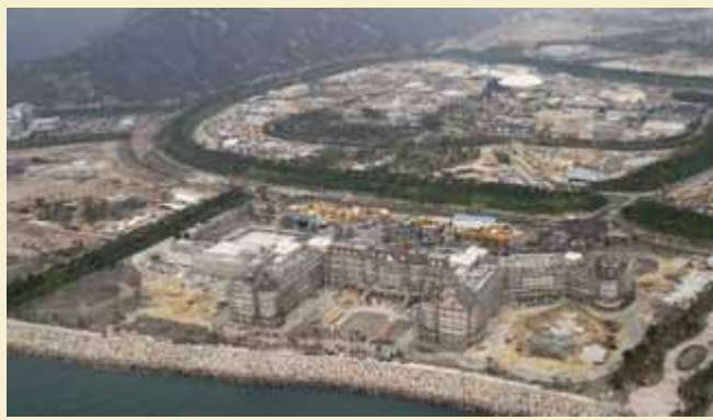
The Hong Kong Disneyland site under construction on Lantau Island.
