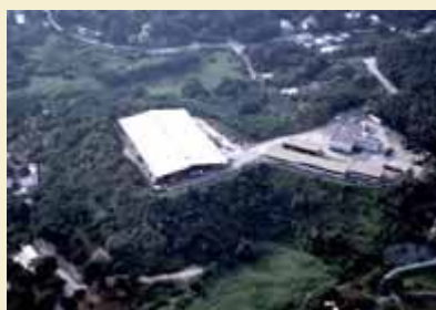
Sha Ling Livestock Waste Composting Plant.
