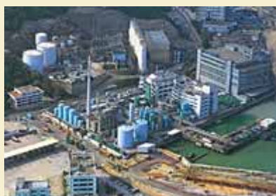
Chemical Waste Treatment Centre, Tsing Yi.
