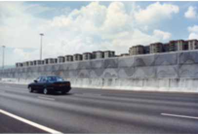
Nearby residents are protected against traffic noise from West Kowloon Expressway through a landscape buffer and noise barriers.
