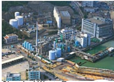
Chemical Waste Treatment Centre, Tsing Yi.
