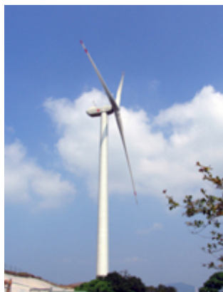
Wind Turbine on Lamma Island.
