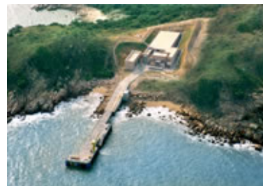
Low-level Radioactive Waste Storage Facility, Siu A Chau.
