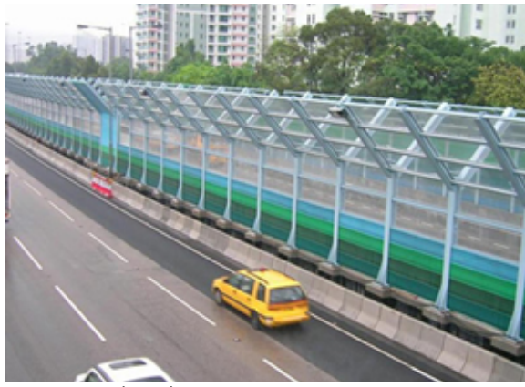
Noise barriers were retrofitted on the Fanling (left) and Sheung Shui (right) sections of Fanling Highway in 2006.
