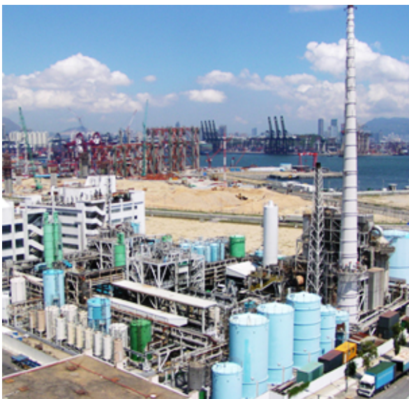
Figure 8 - Chemical Waste Treatment Centre.
