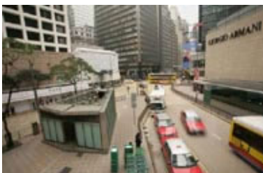
Roadside Air Monitoring Station at Central.
