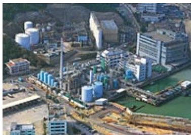
Chemical Waste Treatment Centre, Tsing Yi.
