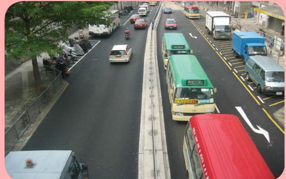
Low noise surfacing at Shek Kip Mei Street
