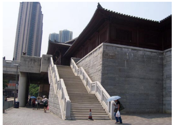
General view at Fung Tak Road
