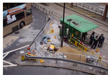
Before near Tram Station (Pennington Street)
