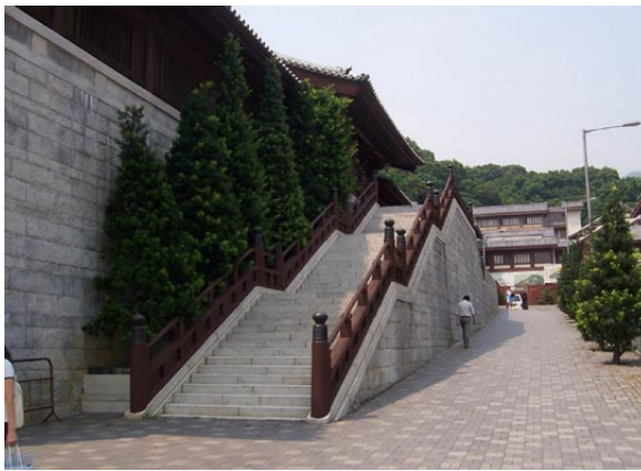
General view at Chi Lin Drive
