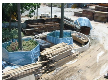
Protection and maintenance of two champion trees within the site area
