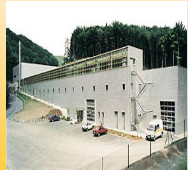
Mechanical-Biological Treatment Plant Asslar
