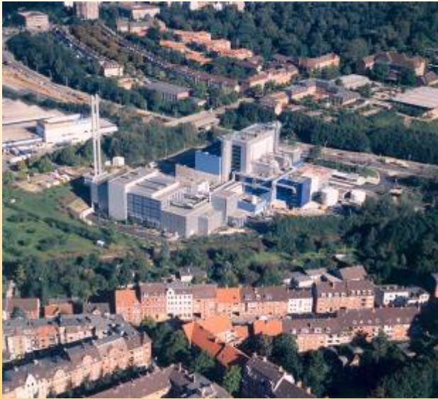
Waste-to-Energy Plant City of Kiel
