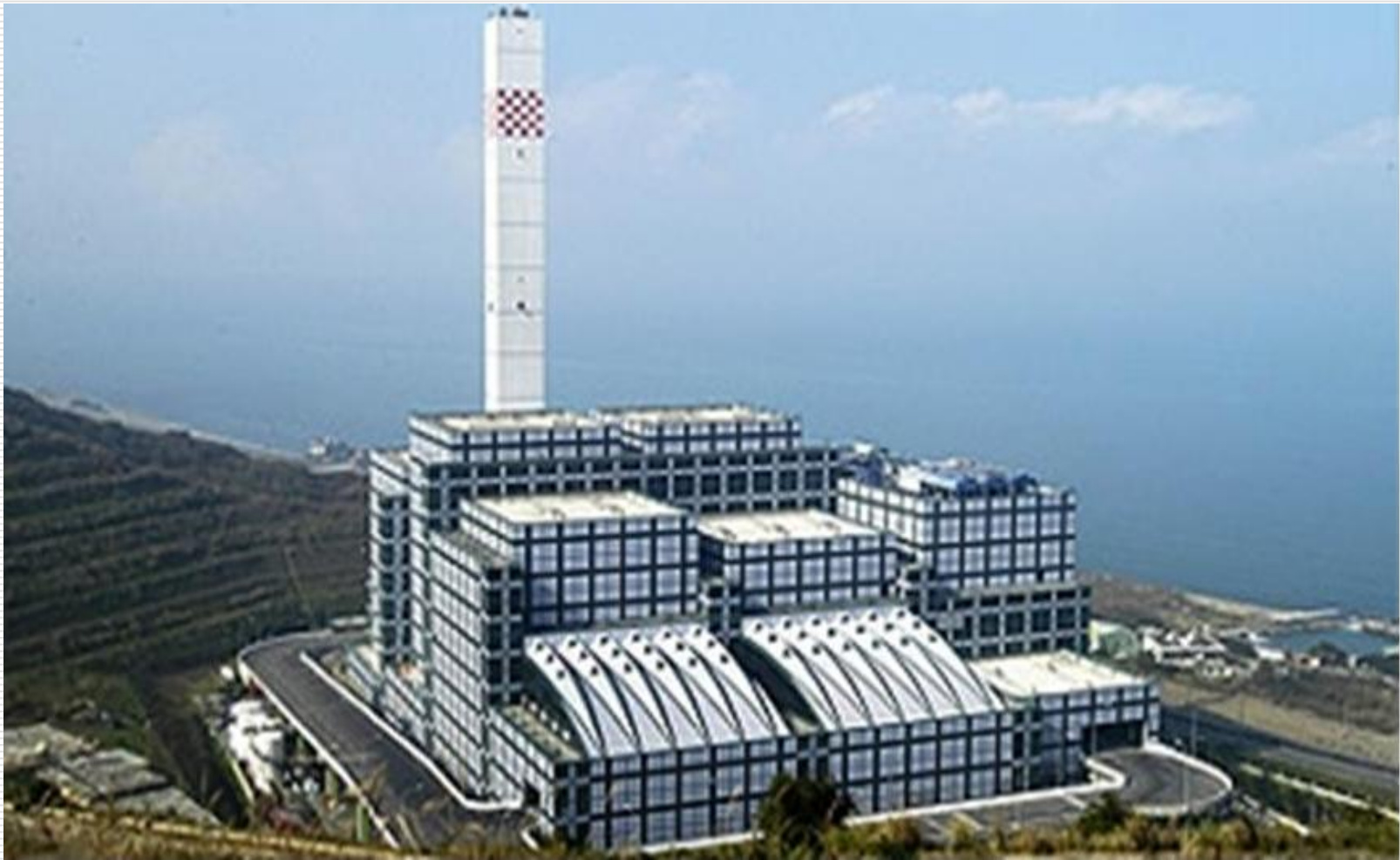
Pa-Li WTE Plant (1,350 mt/day), Taipei County
