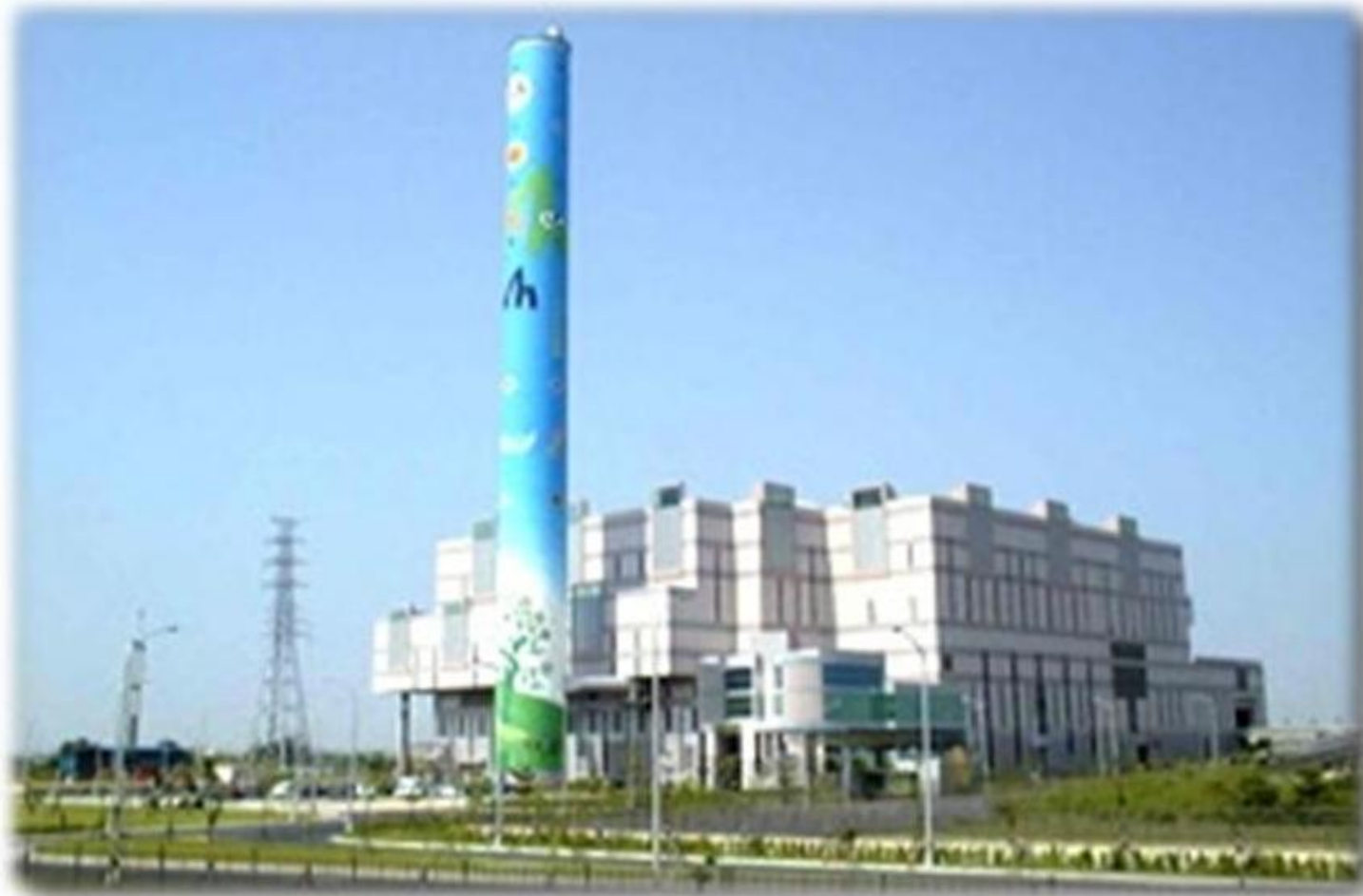
Lu-Tsao WTE Plant (900 mt/day), Chia-Yi County, Taiwan
