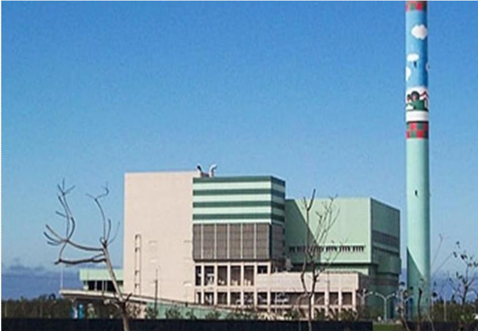
Tainan City WTE Plant (900 mt/day)
