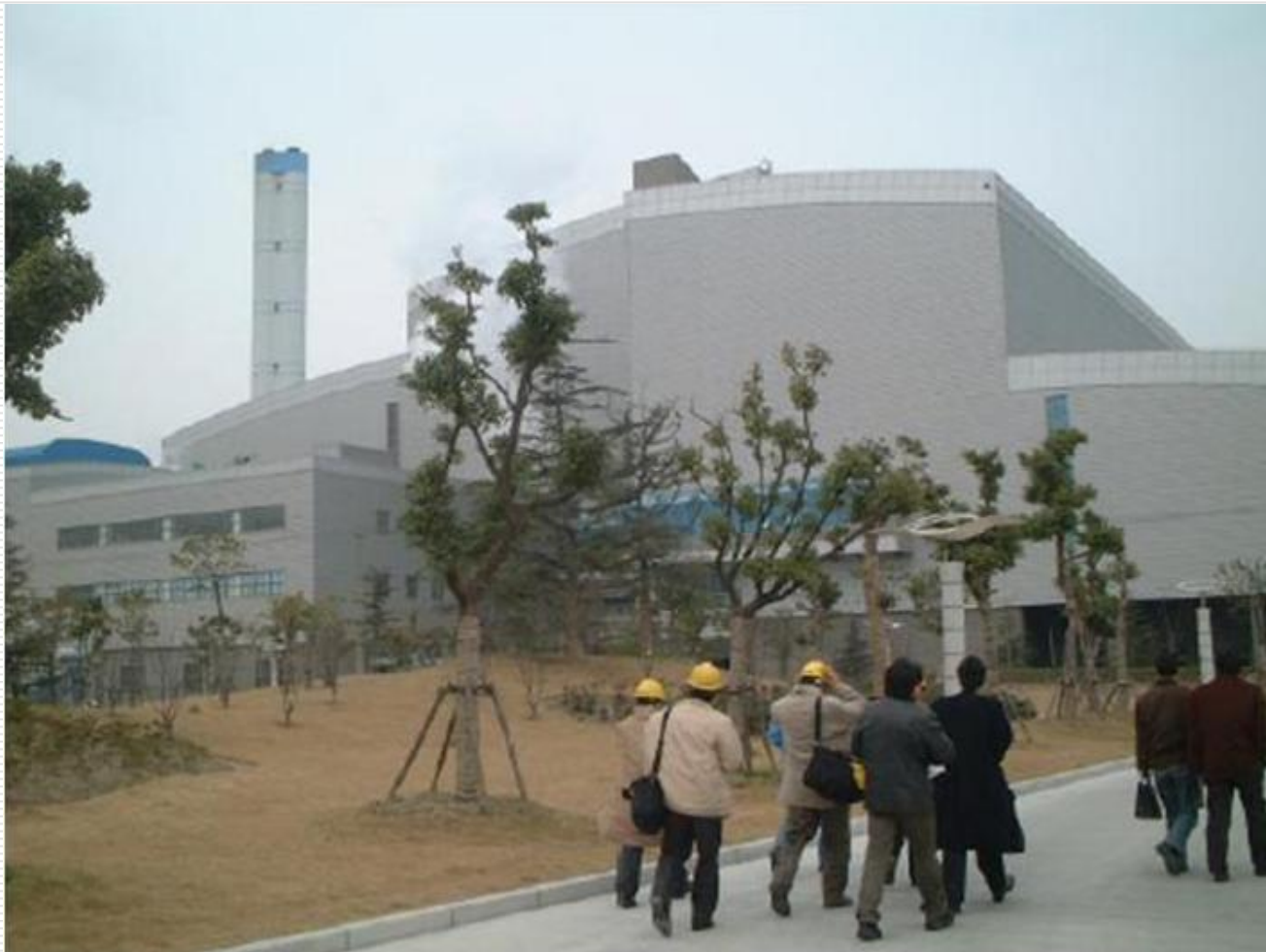
Pu-Xi WTE Plant, Shanghai, China
