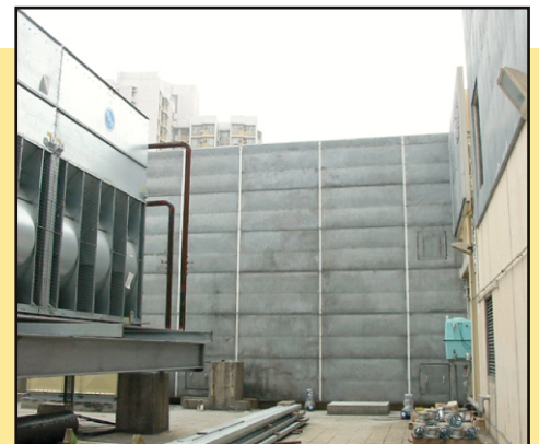
安装隔音屏障以减低对邻近环境的潜在滋扰
