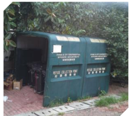
Current Refuse Collection Point in rural area
