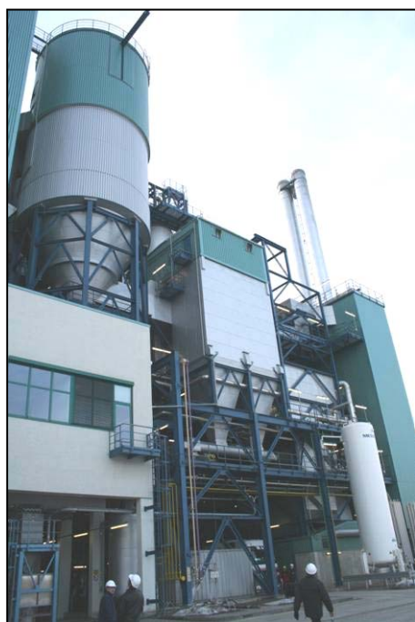
Photo no. 16: The multi-level flue gas purification system and the 55 m chimneys of the T.A. Lauta
