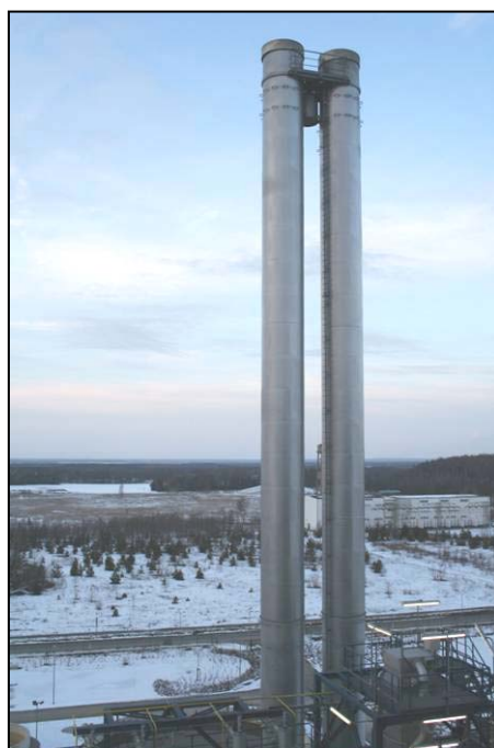
Photo no. 16: The multi-level flue gas purification system and the 55 m chimneys of the T.A. Lauta
