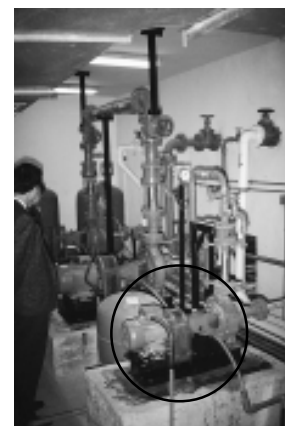
Installation of Isolation Pads (Noise Reduction: 16dB(A))
