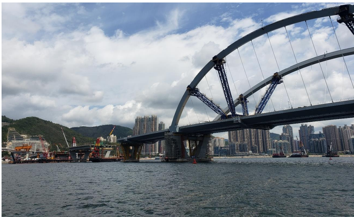
Tseung Kwan O Cross Bay Link under construction across Junk Bay
