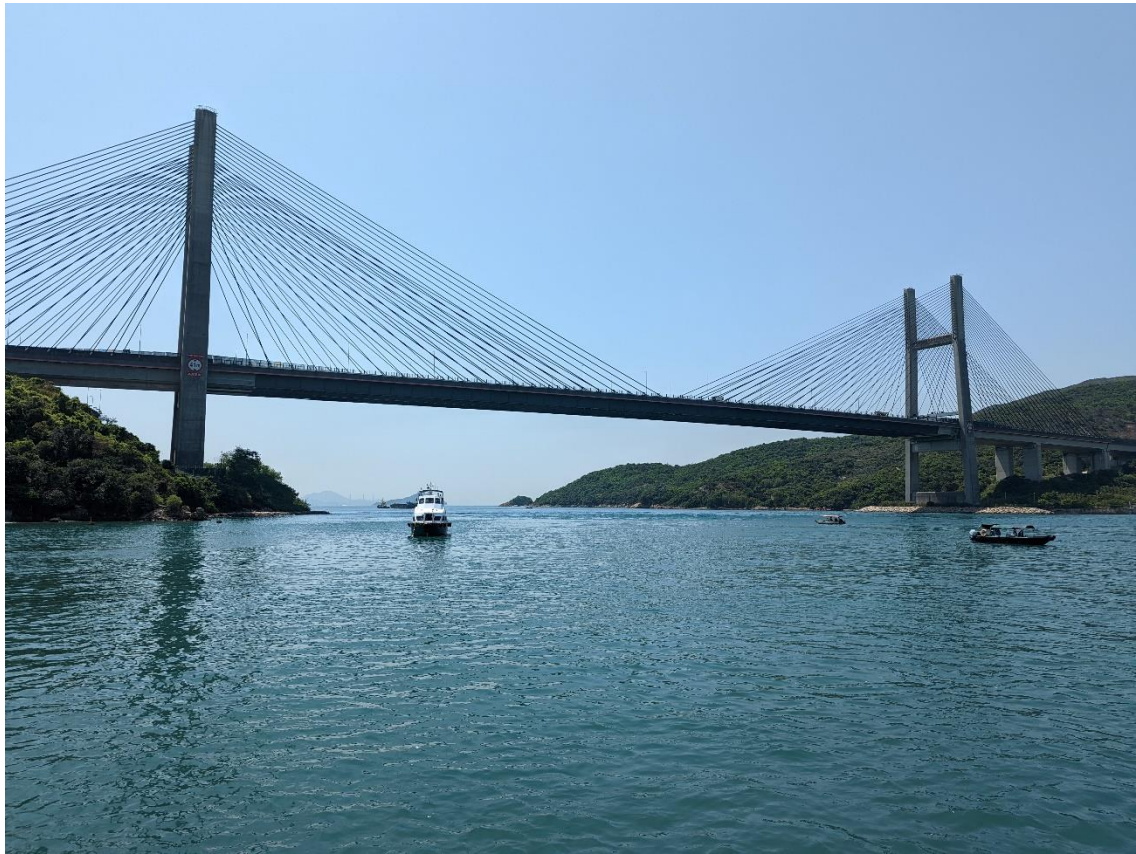
Kap Shui Mun Bridge linking Ma Wan and Lantau Island
