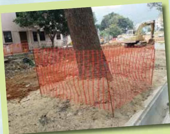
Proper protection of retained trees
