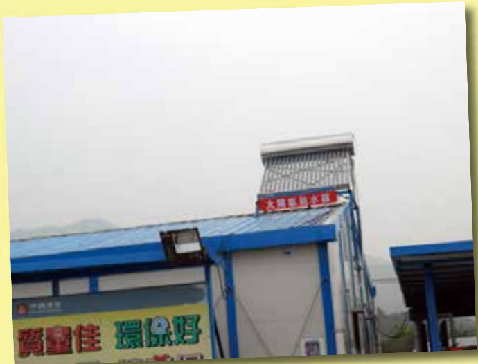
Provision of solar water heater
