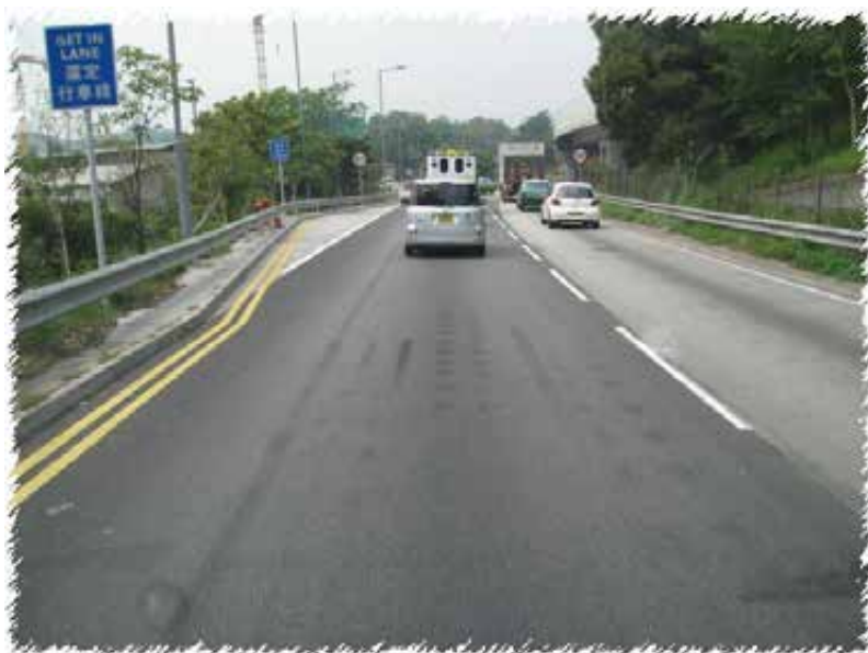
PMSMA surfacing at Pok Oi Interchange, Yuen Long
