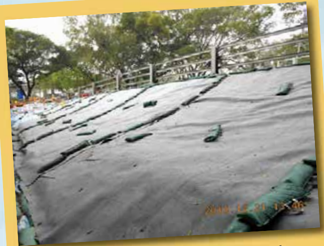
Covering the dusty materials with tarpaulin sheet
