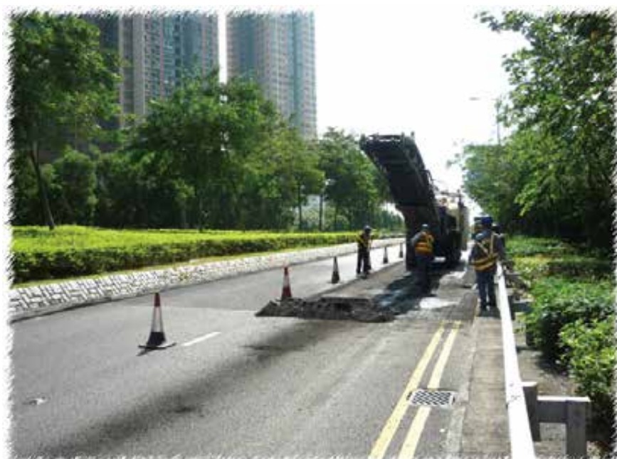
Re-laying PMFC over existing WC
