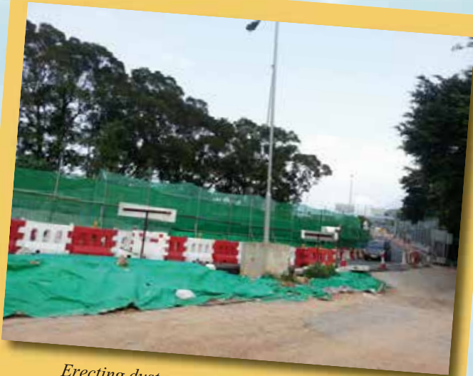
Erecting dust screen alongside works area
