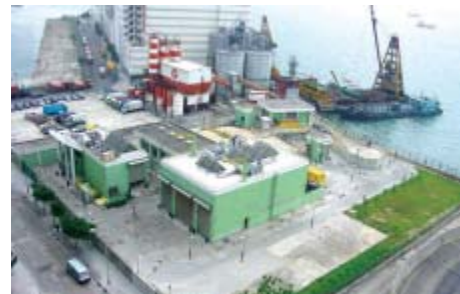
柴灣污水廠的污水已轉流至淨化海港計劃的排污隧道網絡 Sewage from Chai Wan Preliminary Treatment Works has been diverted to the tunnel network of HATS
