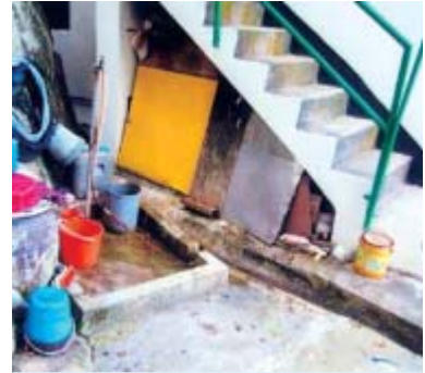
生活污水可經地面明渠流入水道 Sullage can be discharged via surface channels to watercourses
