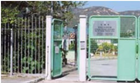
建議中會擴充梅窩污水處理廠以處理來自南大嶼山的污水 The upgrading of Mui Wo STP has been proposed to treat also the flow from the south of Lantau
