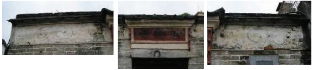
Façade Wall Frieze Decorative Feature of the Fourth Bay from the Easternmost End
