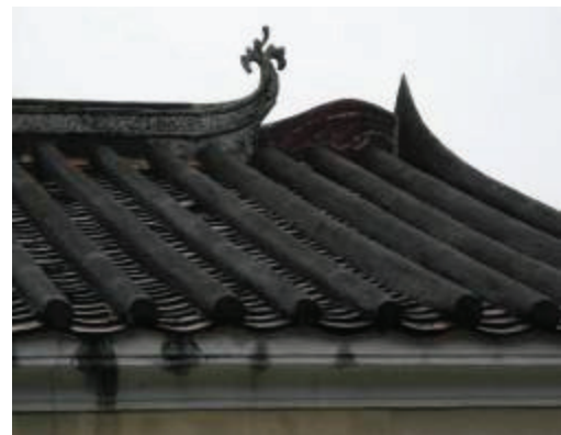
Boat Shape Rear Roof Ridge
