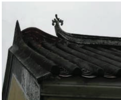
Boat Shape Rear Roof Ridge
