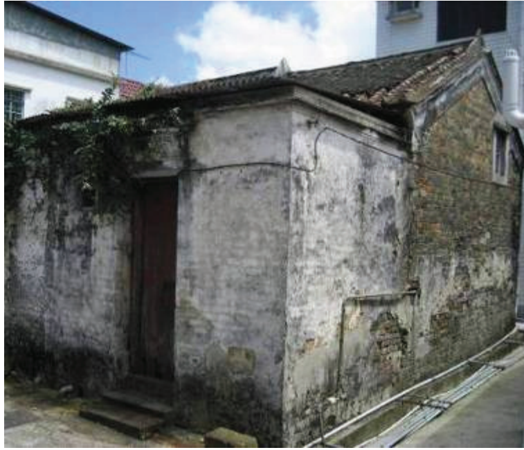
General Front View of West Bay and West Side Wall
