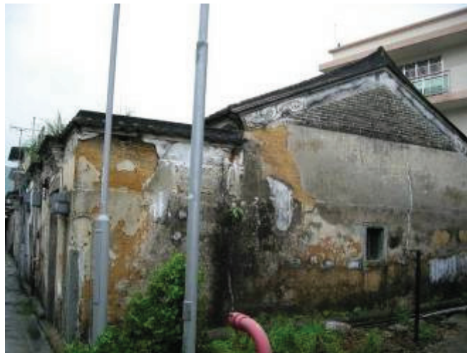
West Side Wall with Window Opening
