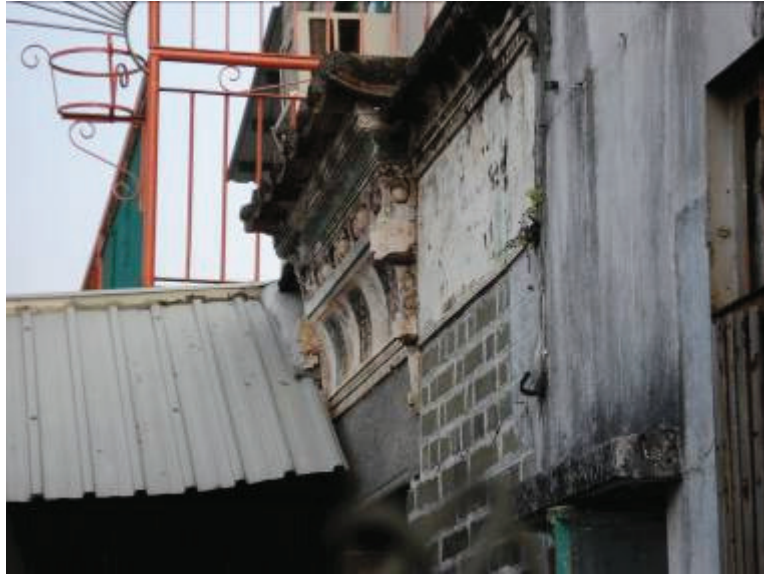
Decoration above Lintel of No. 40 Tsung Yuen Ha
