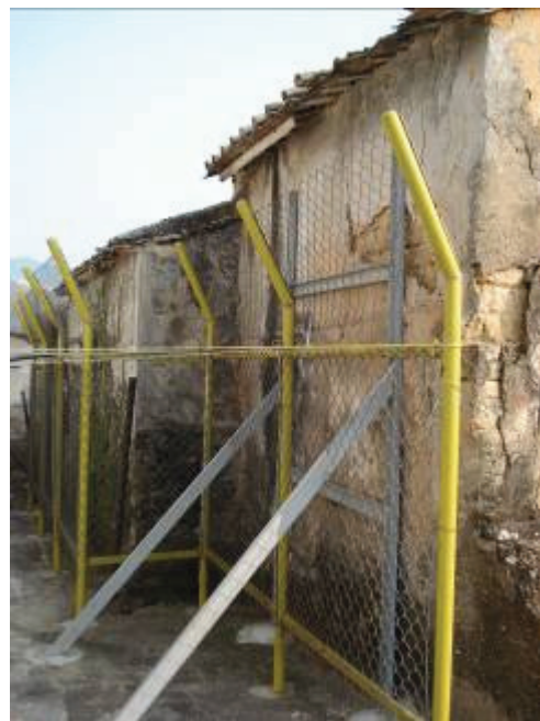
Back View (With External Structural Support)
