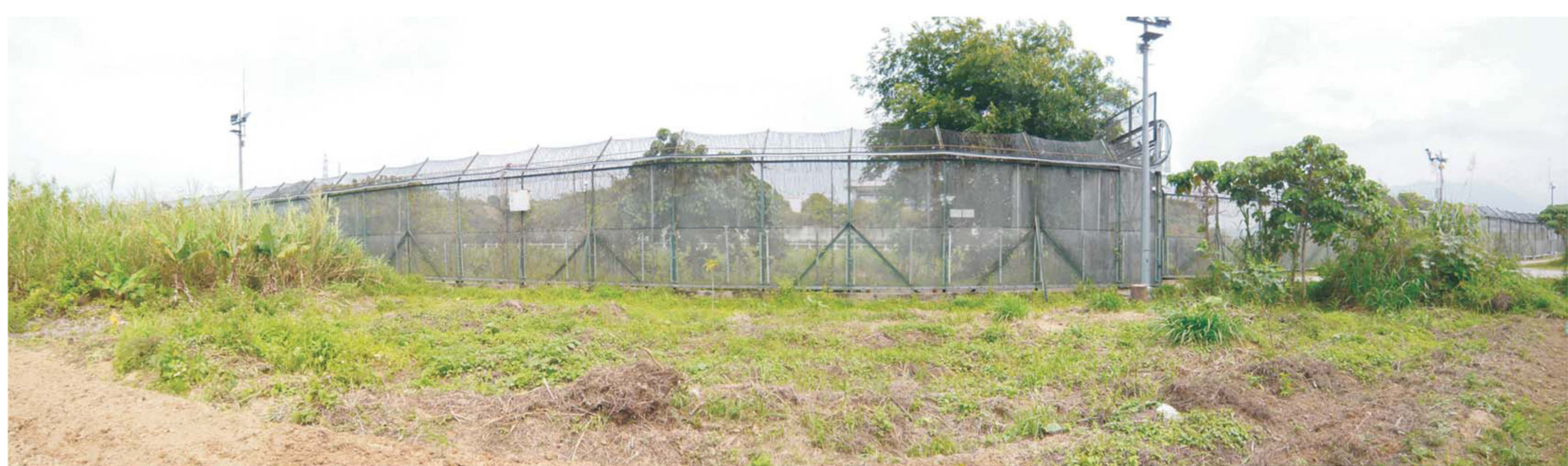
Existing view from Ta Kwu Ling Village Towards the Project Site
