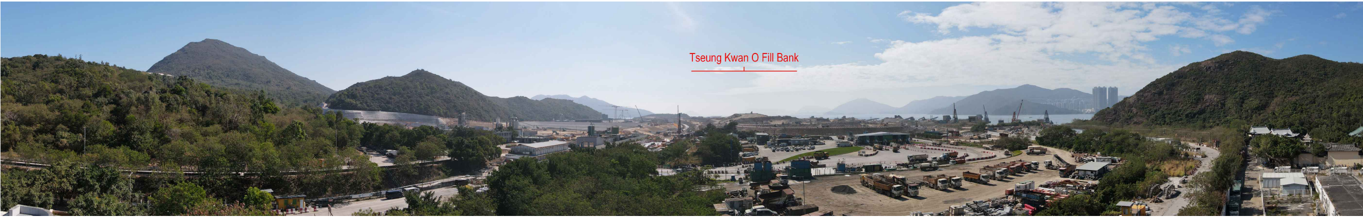
VSR3 - TVB Broadcast and Production Centre
