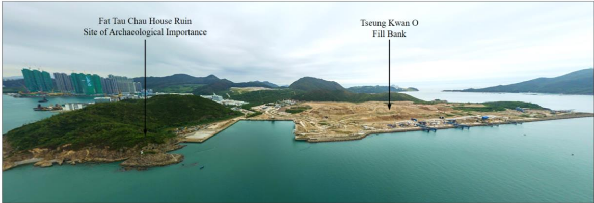
Figure 9.1 Location of Fat Tau Chau House Ruin SAI and TKOFB
