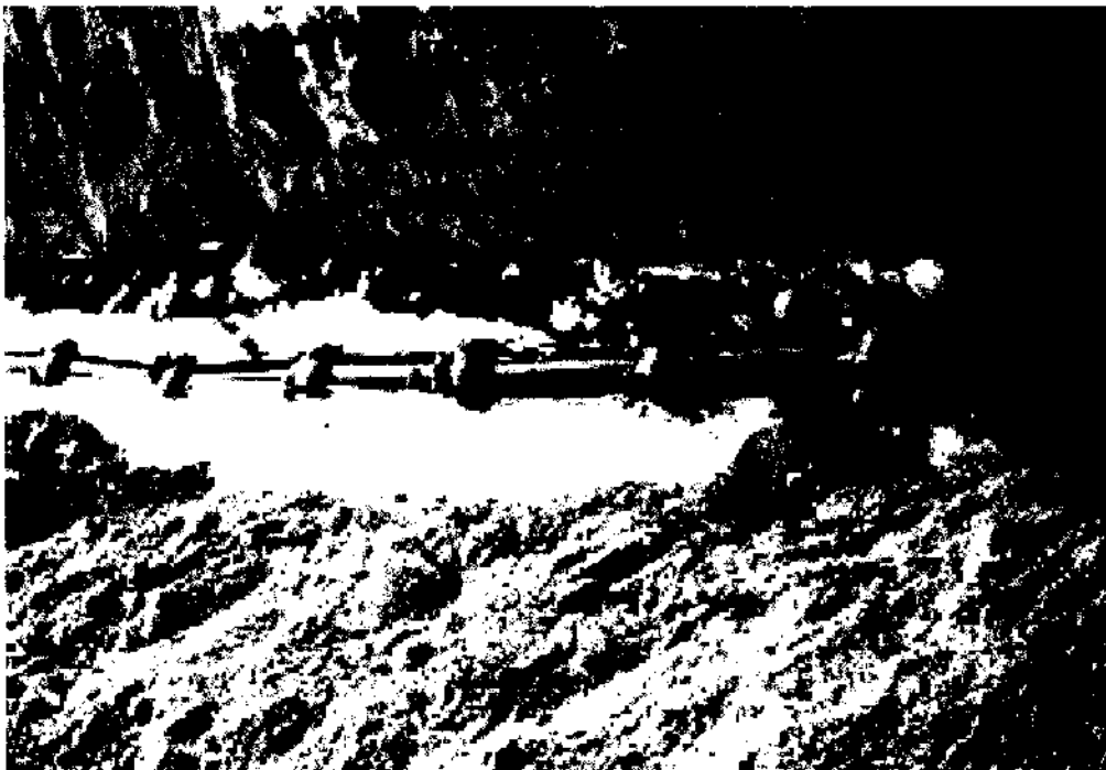
FIGURE 7 - CABLE FITTED WITH ARTICULATED PIPES
