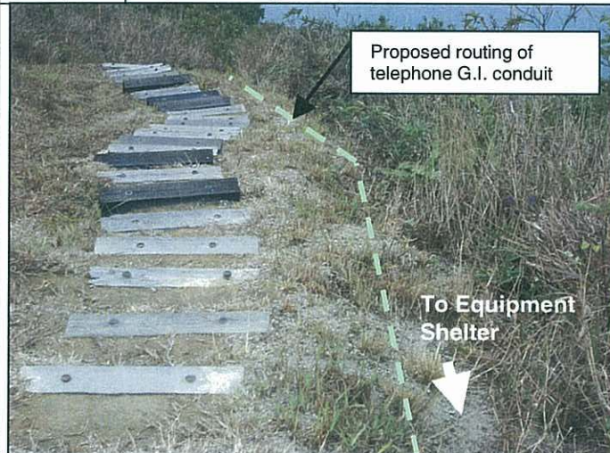
Photo No. 11 Location Ling Kok Shan Description Proposed routing of telephone G.I. conduit
