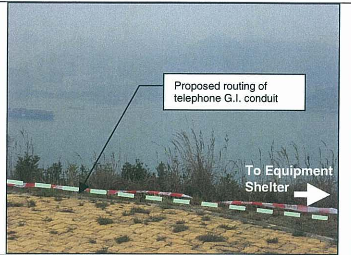
Photo No. 8 Location Ling Kok Shan Description Proposed routing of telephone G.I. conduit
