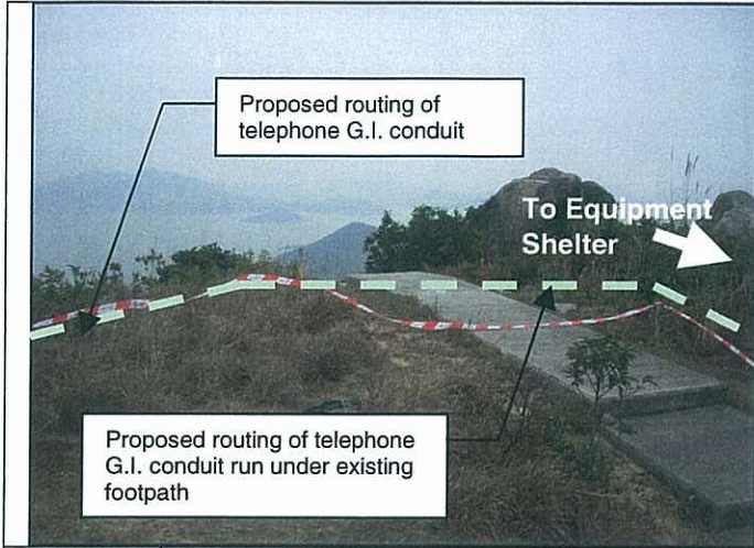
Photo No. 7 Location Ling Kok Shan Description Proposed routing of telephone G.I. conduit
