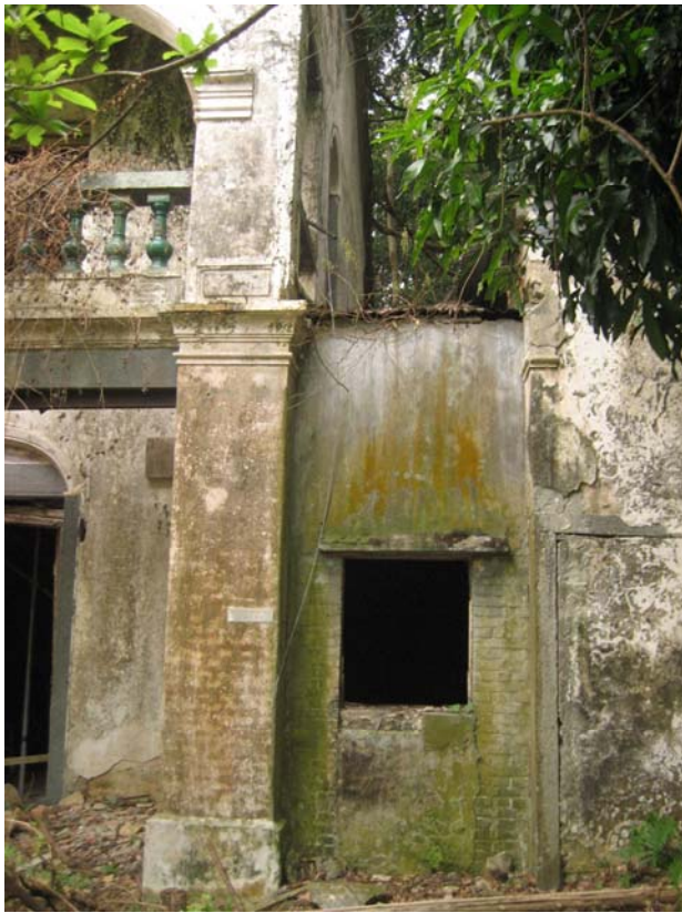
Photo 5 Aisle Connecting the Main Building and the Annex Block 相片 5 連接主樓和附建物之通道
