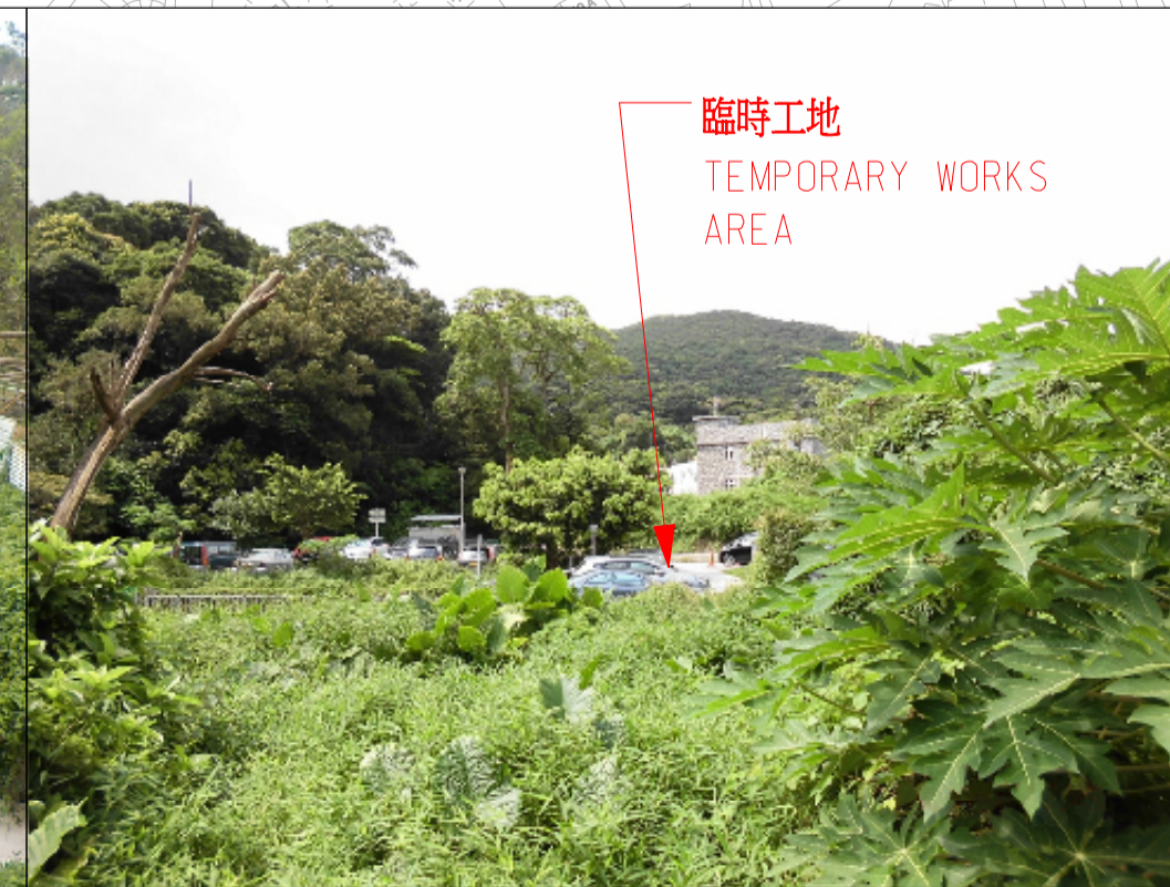
從VSR4望向臨時工地 VIEW OF THE TEMPORARY WORKS AREA FROM VSR 4
