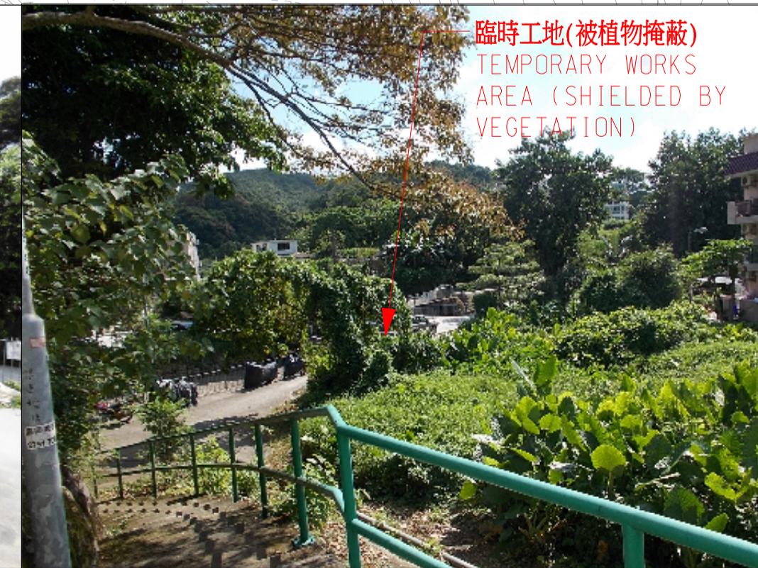
從VSR6望向臨時工地 VIEW OF THE TEMPORARY WORKS AREA FROM VSR 6
