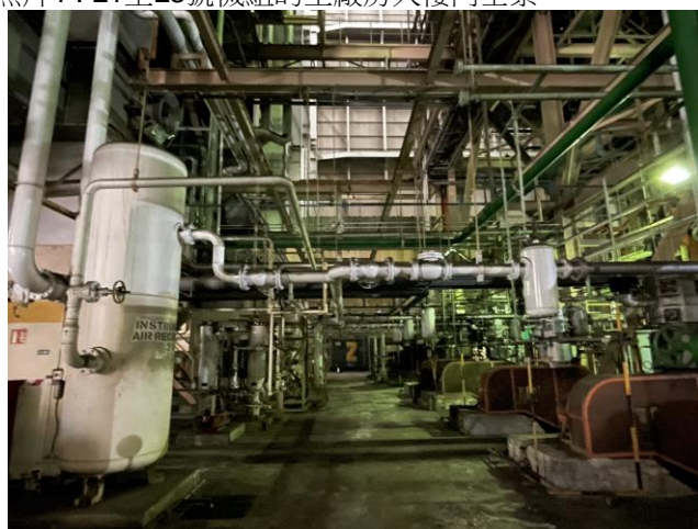
Photo 4: Overall view inside the Main Station Building for L1 to L3
