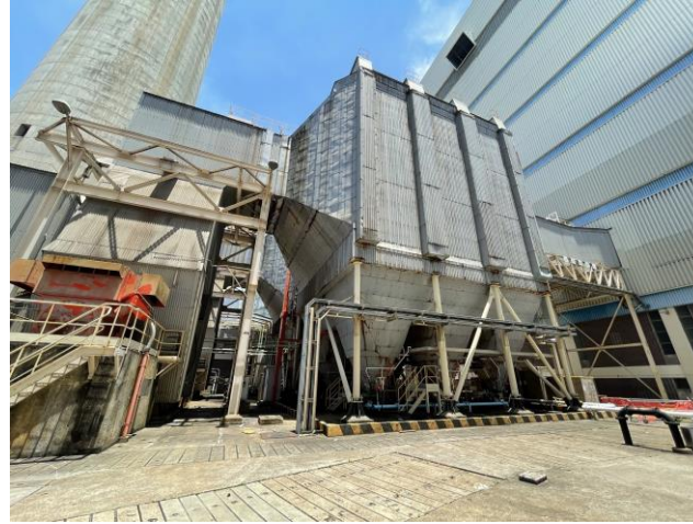
Photo 62: Electrostatic precipitator systems connecting from the Main Station Building for L1 to L3 照片 62：連接L1至L3號機組的主廠房大樓的靜電除塵系統
