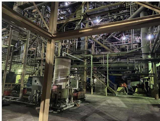
Photo 2: Overall view inside the Main Station Building for L1 to L3
