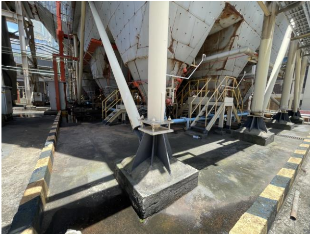
Photo 64: Ash hopper of the electrostatic precipitator system 照片 64：靜電除塵系統的煤灰漏斗
