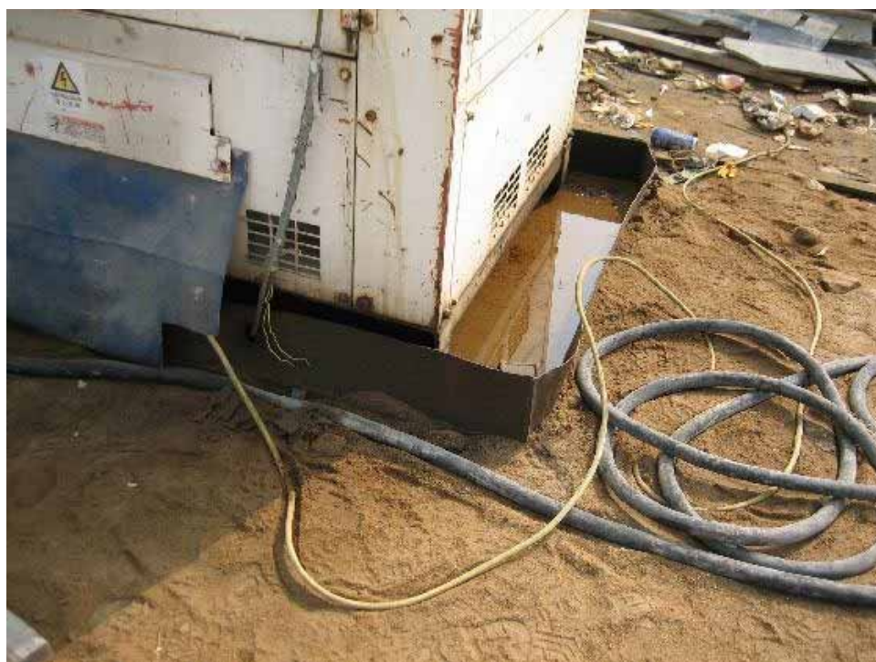
Fig. 1 Drip tray leakage was repaired.
