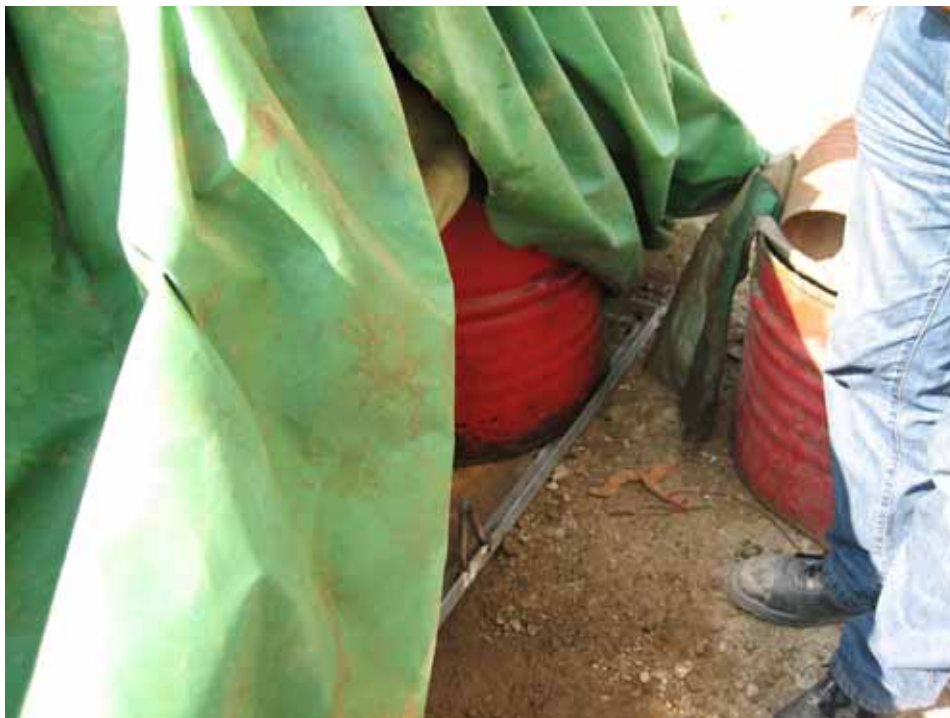
Fig. 4 Drip trays has been provided for the chemical drums near the chemical drum storage cabinet.
