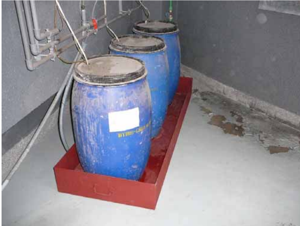
Fig. 2 Drip pan is provided for the three plastic chemical drums adjacent to the cooling tower in the administration building.
