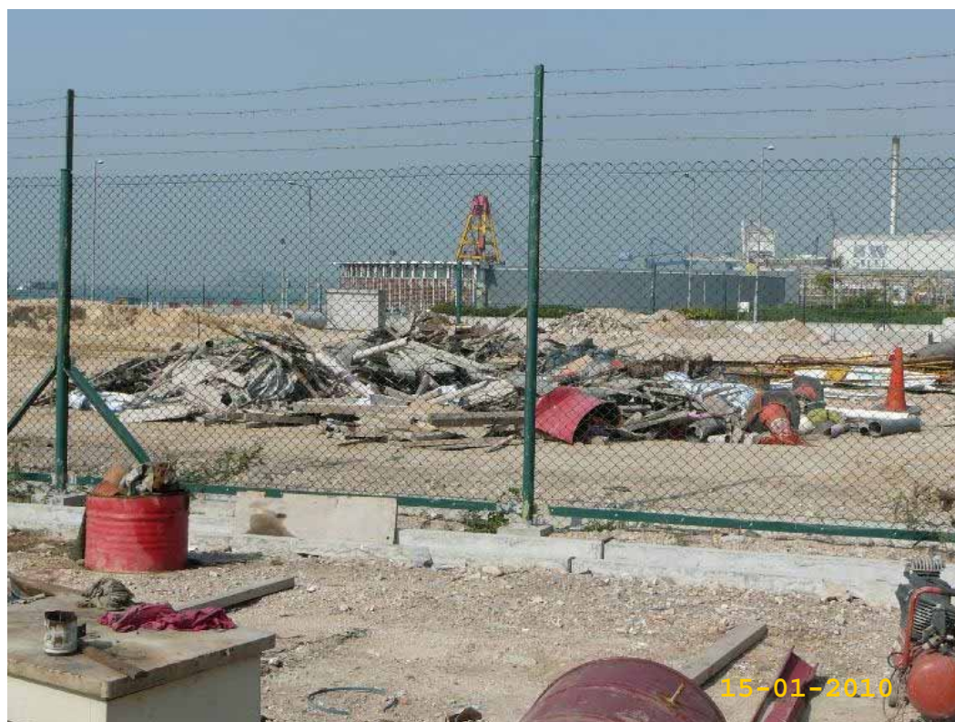
Fig. 2 Piles of waste wood and boards were temporarily stored at centralized collection location for further disposal from the site.
