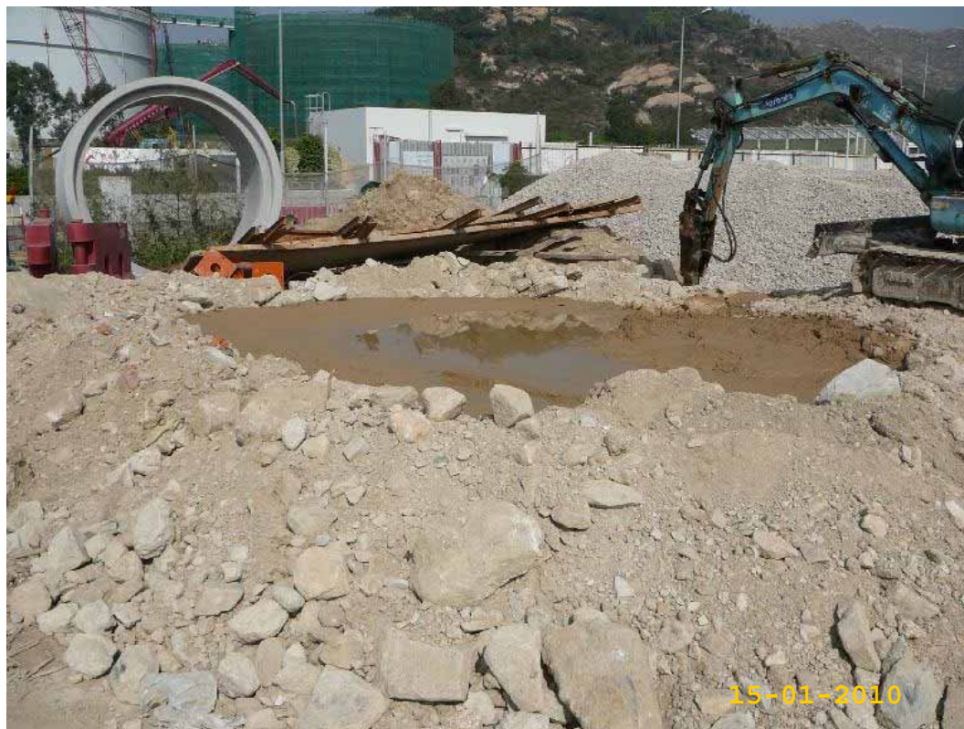
Fig. 8 Contaminated concrete and soil was removed.
